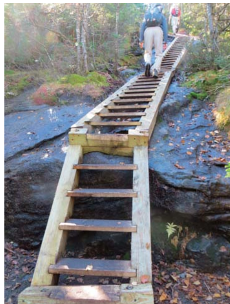
Trail rehabilitation on Mt Colden sup- ported by 46er contributions
